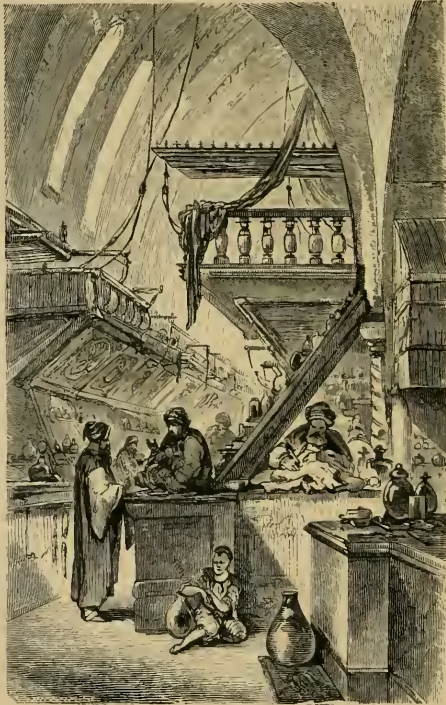
A PERFUME BAZAAR IN THE EAST
